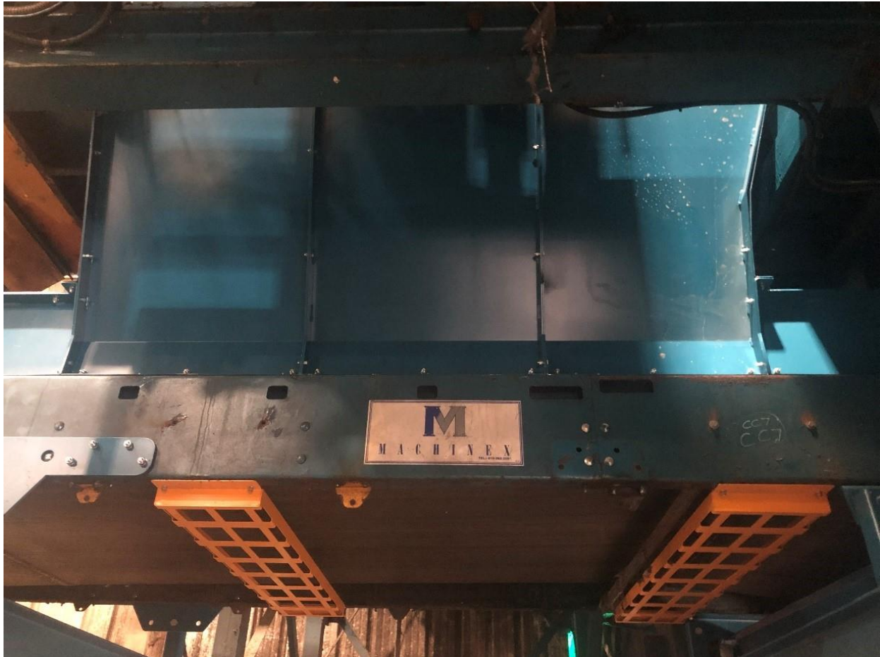
Figure 1 – New Chutes and Repositioned Existing Conveyor
