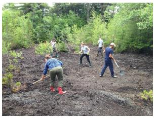
Figure 7. Hand spreading of compost in Northern end of Wildcat Shale Pit Remediation site.
