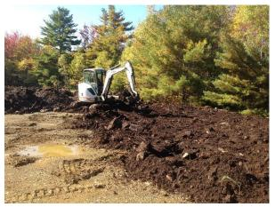
Figure 6. Spreading and landscaping with excavator in Western side of Wildcat Shale Pit Remediation Site.
