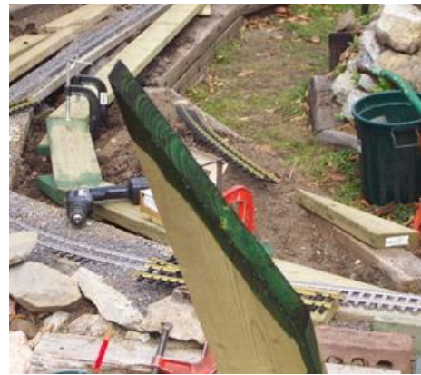
Figure 2.7 Wood with Preservative Applied
