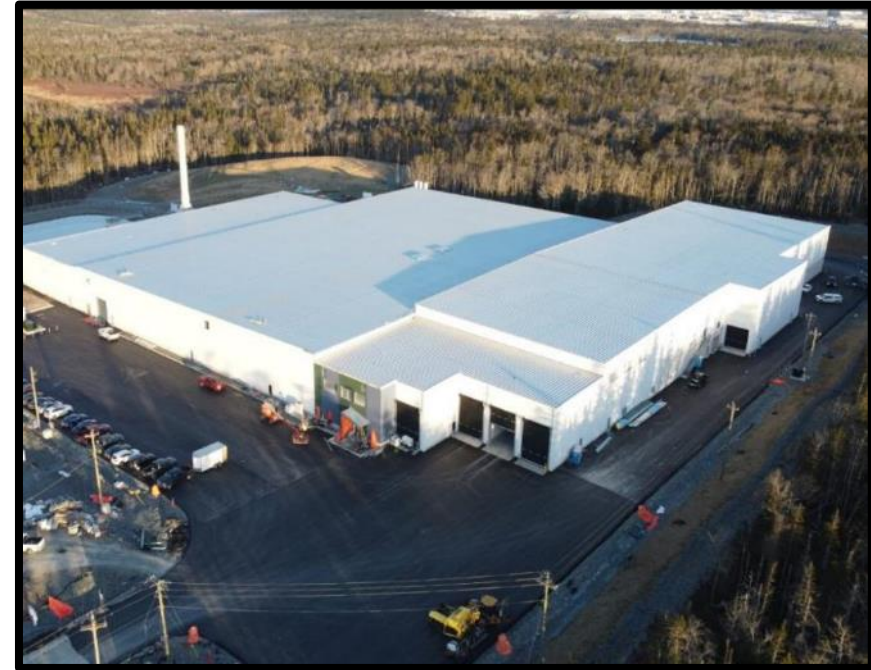
New Ragged Lake Organics Facility, Photo: HCR
