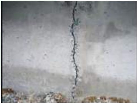
Foundation Crack Repairs
